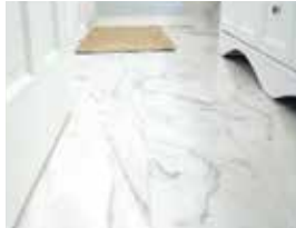
Zenith A2, DSC Installing porcelain tile with the continuation of texture patterns
